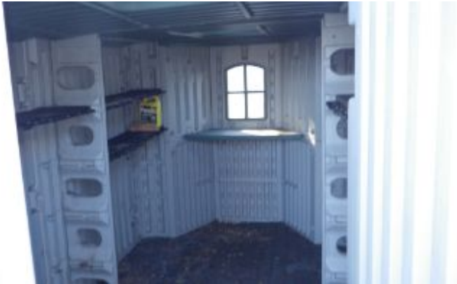
PVC Shed observed in rear of property
