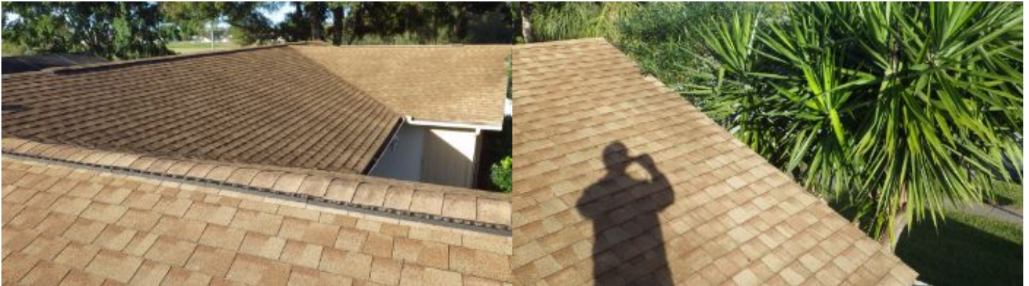
The county records indicate that the roof was replaced in 2006.
