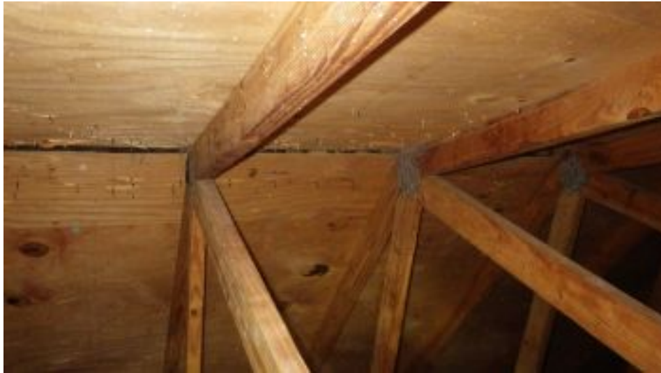
All visible areas clean and dry, except as noted
