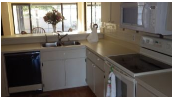
Kitchen cabinets, appliances, fixtures, lighting and counters appear sound and clean except as noted.
